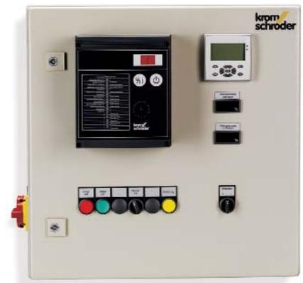
Fig. 9: Control cabinet for a cascade control system for a single burner
